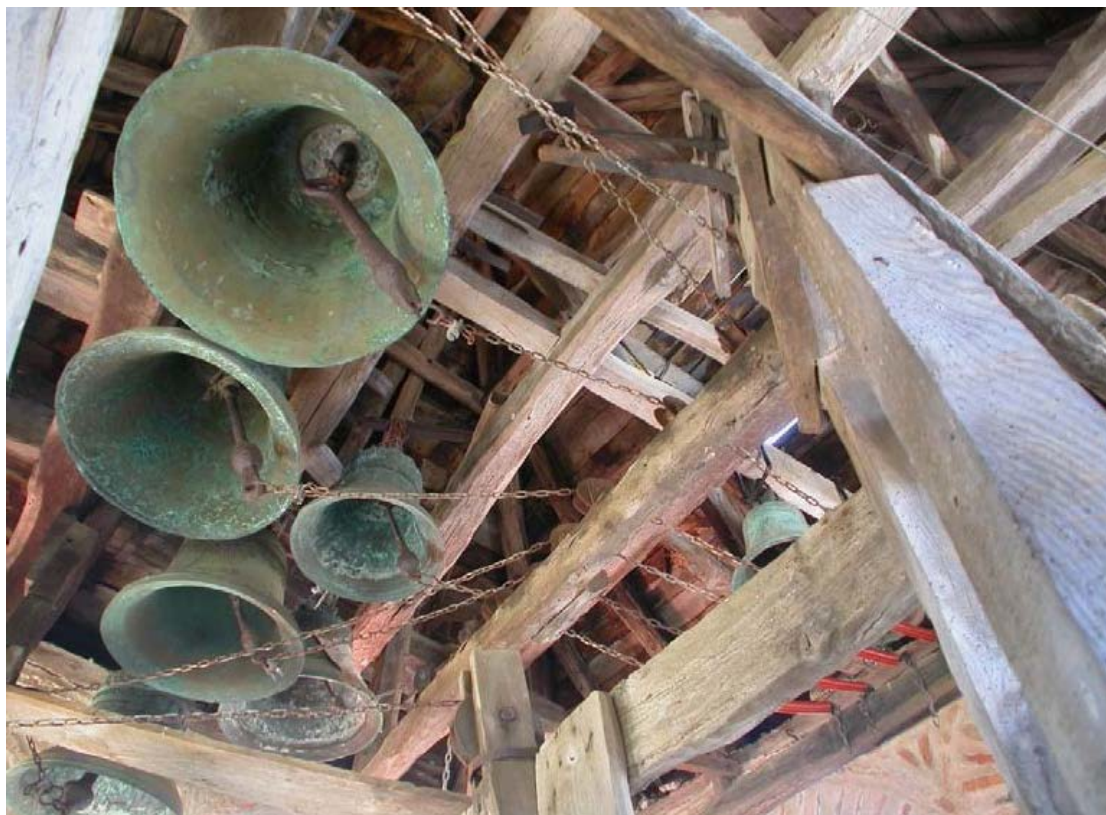
PICTURE 3 – DAMAGE TO THE WOODEN STRUCTURE CAUSED BY DAMP
