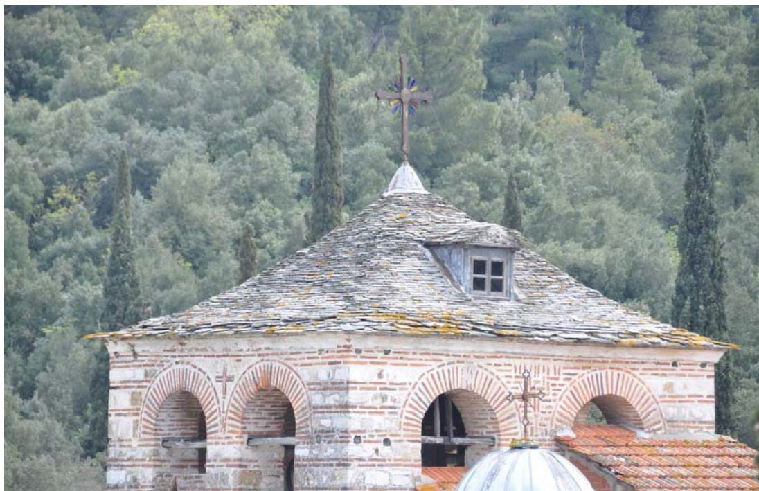
PICTURE 1 – VIEW OF THE BELL TOWER’S ROOF
