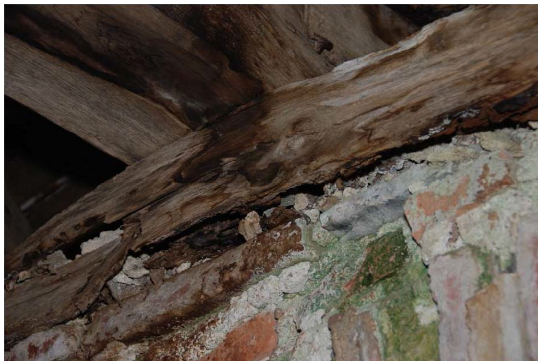
PICTURE 3 – DAMAGE TO THE WOODEN STRUCTURE CAUSED BY DAMP
